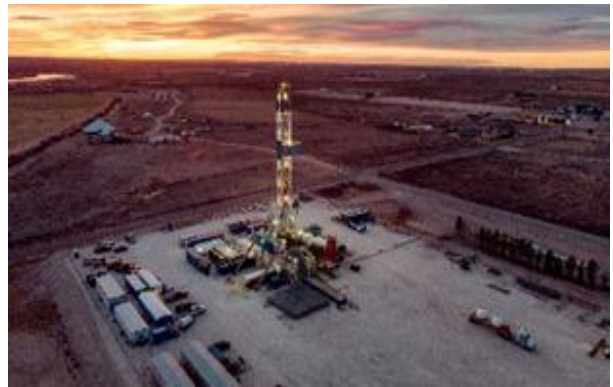
Figure 4 Typical piping and pad site setup
